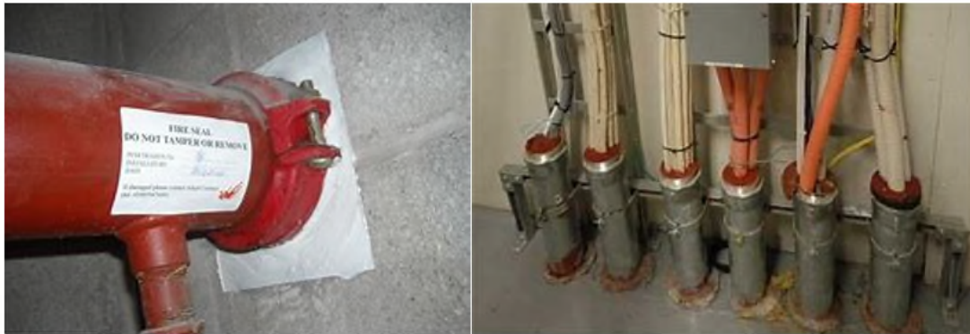
Figure 4: Fire Stopping Through Walls and Floors
